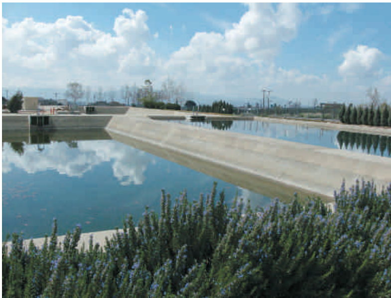
Treatment Plant 134, a surface water treatment plant located at Highland Avenue near the 330 Freeway, is subject to new governmental regulations and must convert to a membrane micro-filtration facility by 2012.
