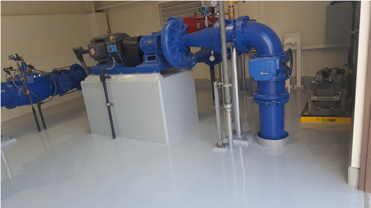
Exhibit 1: One of two hydroelectric generation units at Plant 134.
